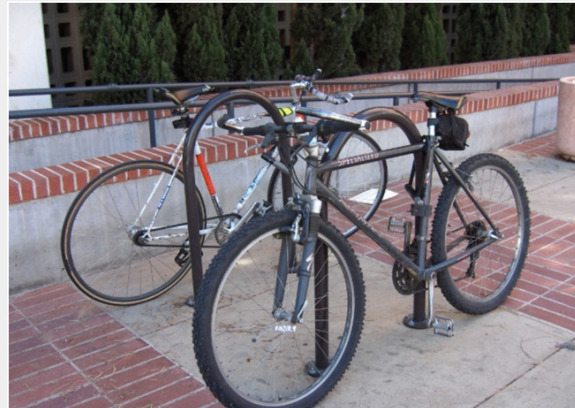
FIGURE 3.3.2 – INVERTED U BIKE RACK
